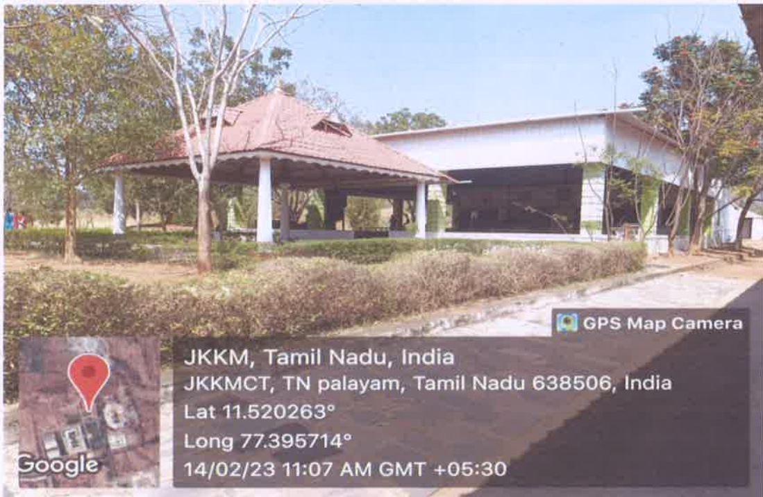
FIG 36: CANTEEN-I OUTSIDE VIEW
