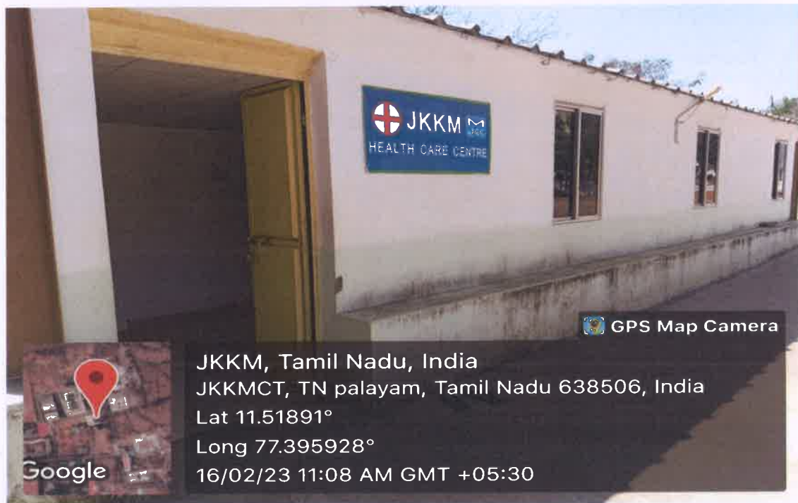
FIG 20: HEALTH CENTRE OUTSIDE VIEW
