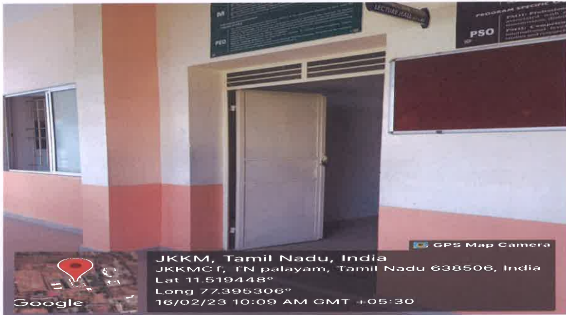
H-305 Classroom outside view
