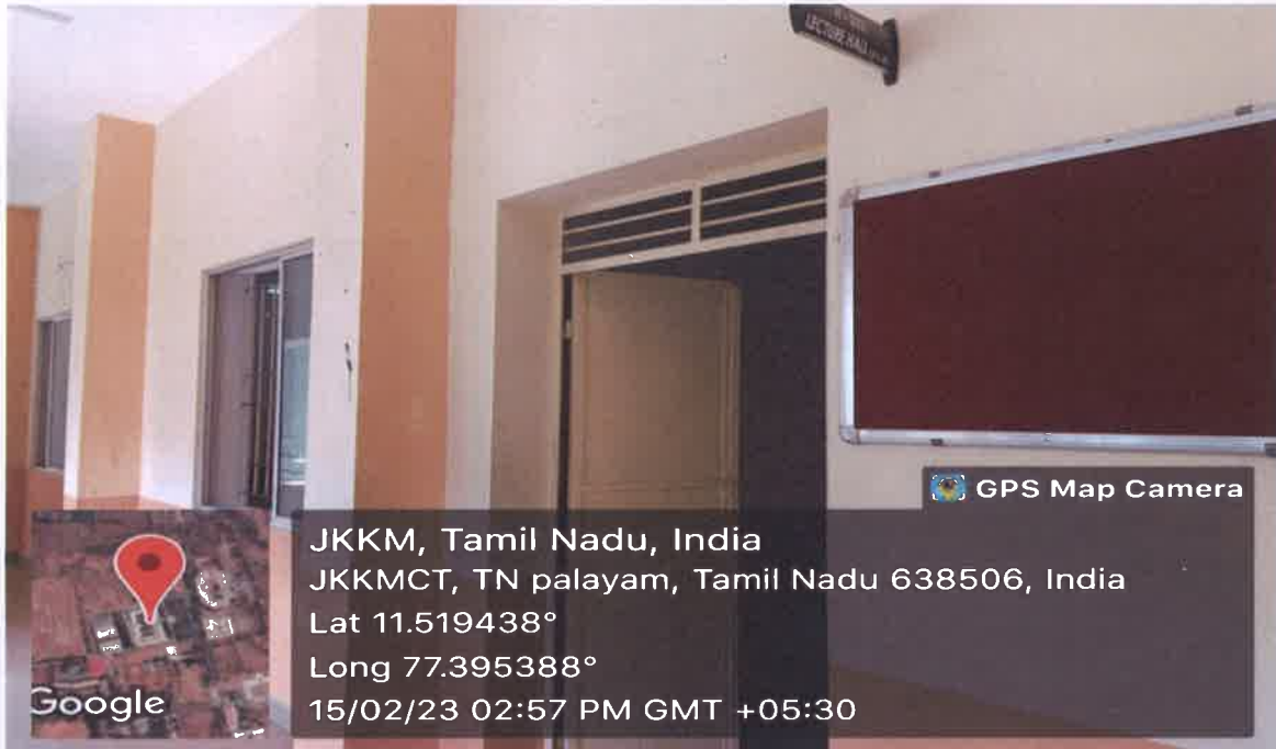
H-202 Classroom outside view
