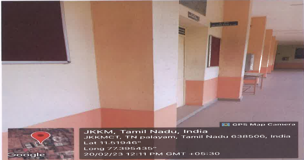
H-414 Classroom outside view
