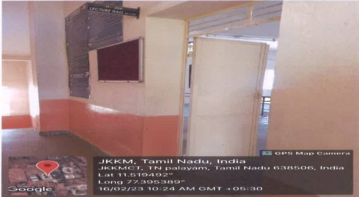
H-208 Classroom outside view
