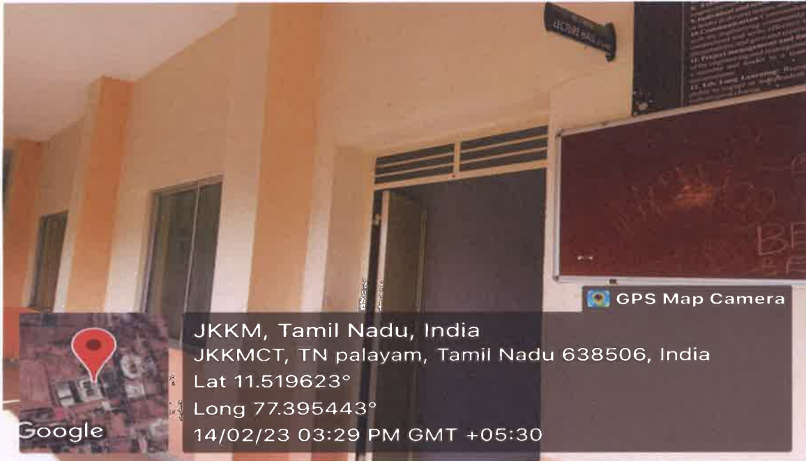
H-410 Classroom outside view
