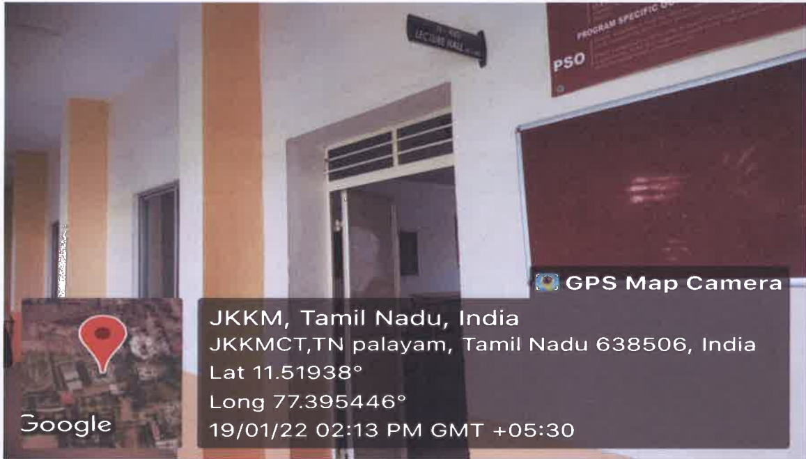
H-420 Classroom outside view
