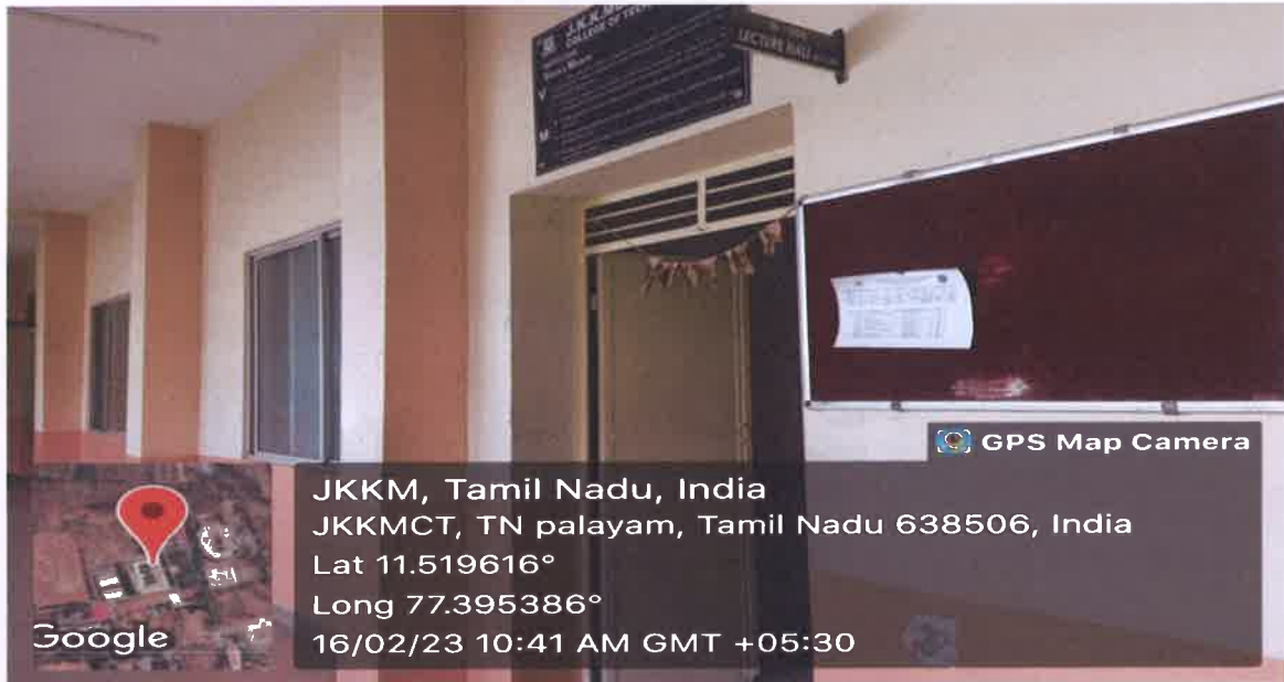
H-206 Classroom outside view
