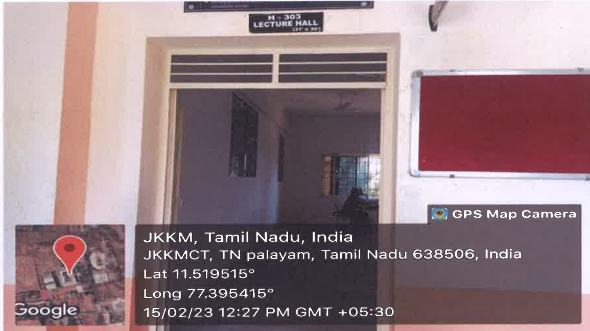
H-303 Classroom outside view
