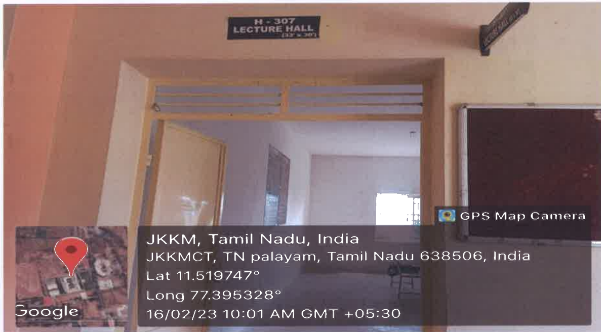
H-307 Classroom outside view
