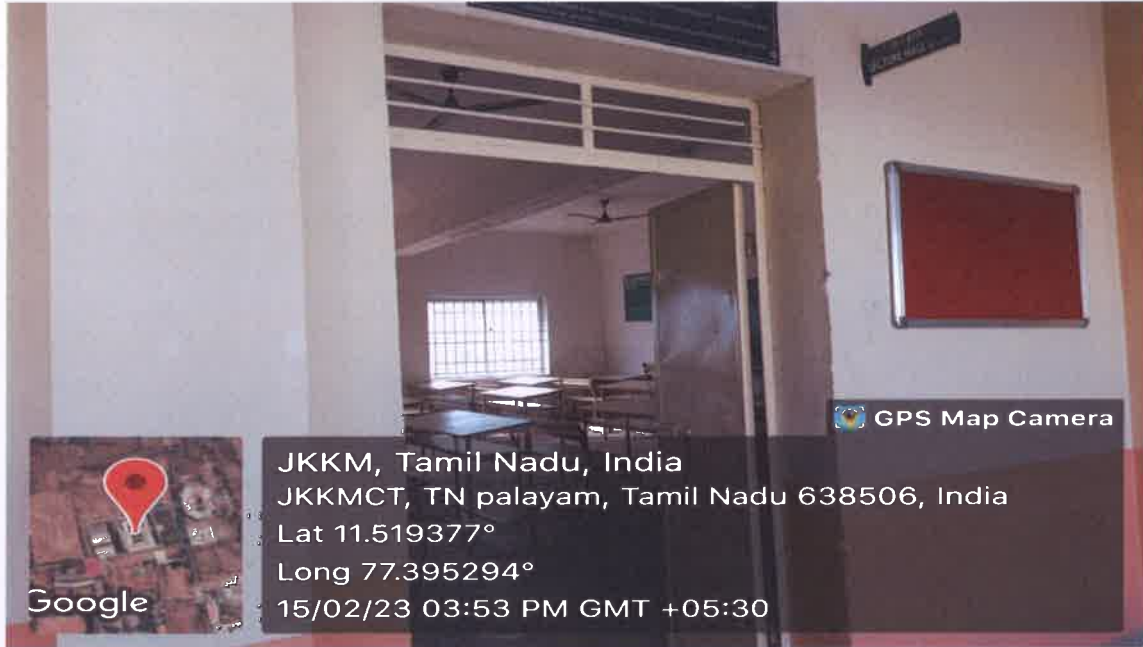
H-418 Classroom outside view
