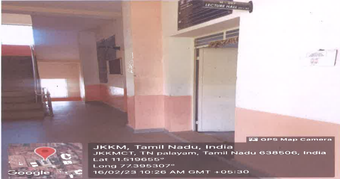
H-207 Classroom outside view
