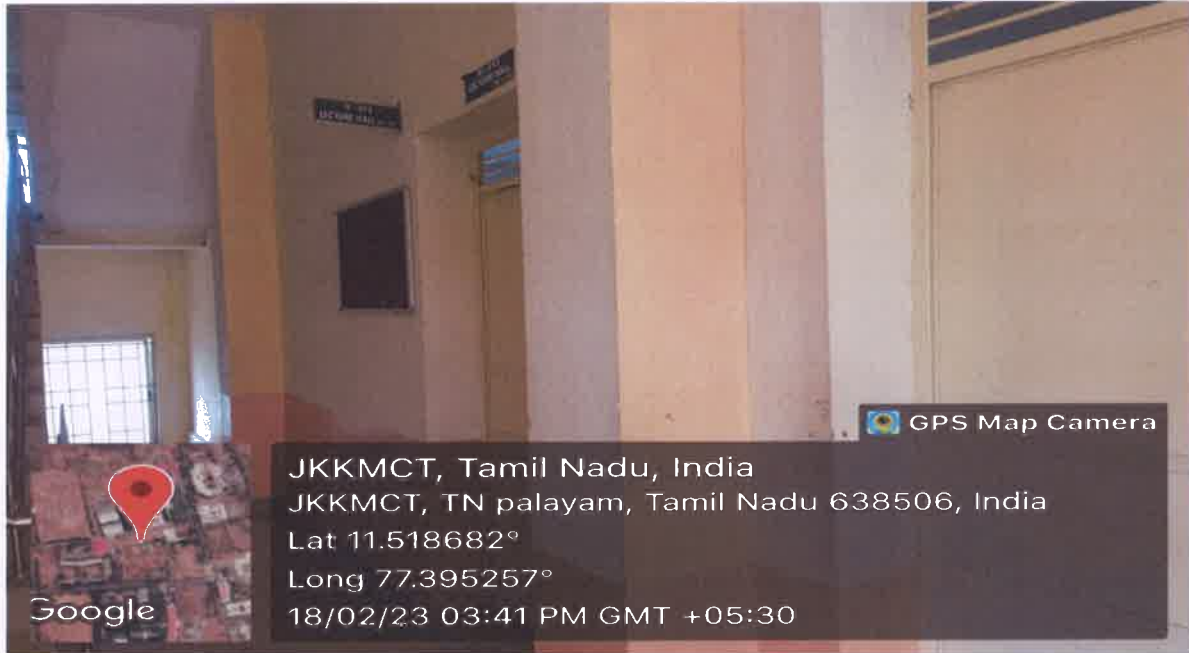
H-412 Classroom outside view
