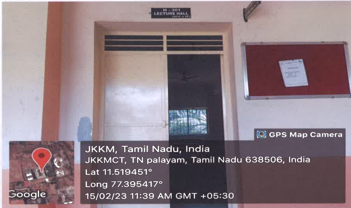
H-301 Classroom outside view
