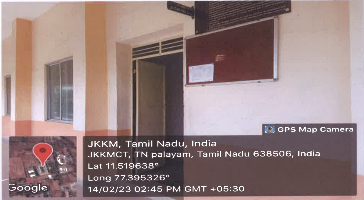
H-409 Classroom outside view
