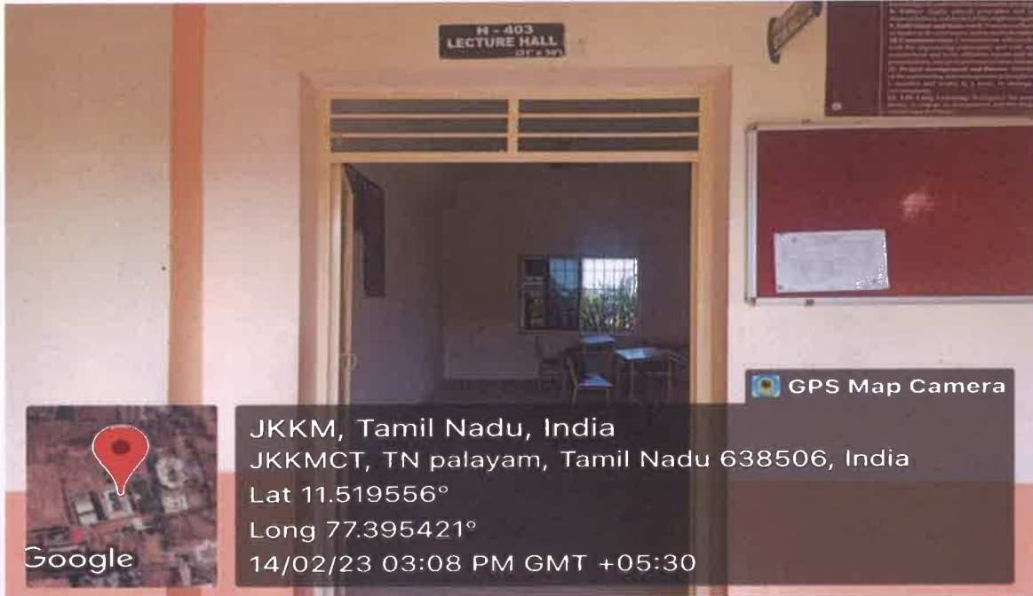
H-403 Classroom outside view
