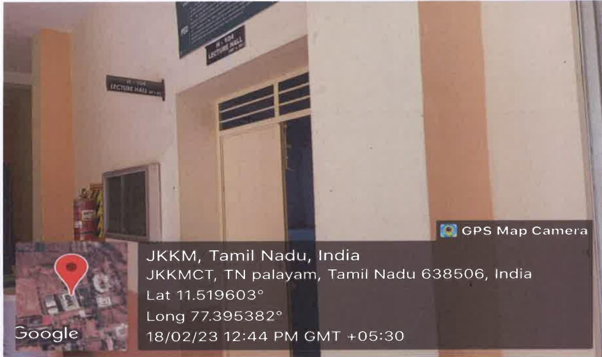
H-104 Classroom outside view
