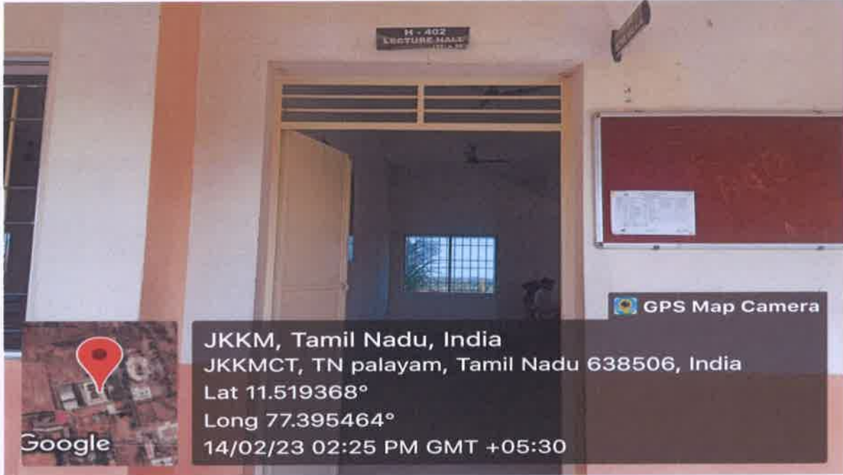
H-402 Classroom outside view
