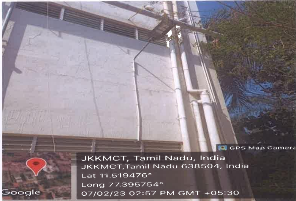
Photo of Sensor based automatic light located near Basketball ground
