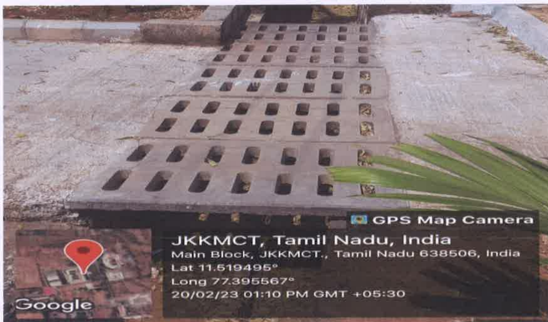
Photos of Distribution system in the campus
