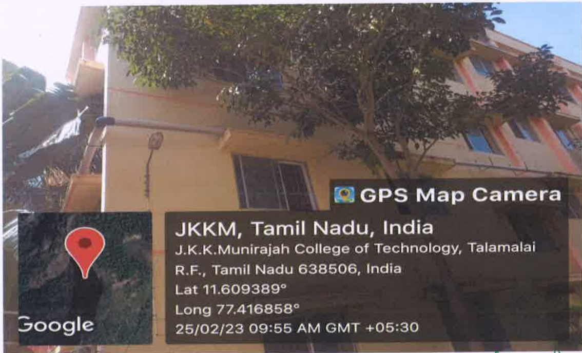
Photos of Rain water pipe lines in Main Block
