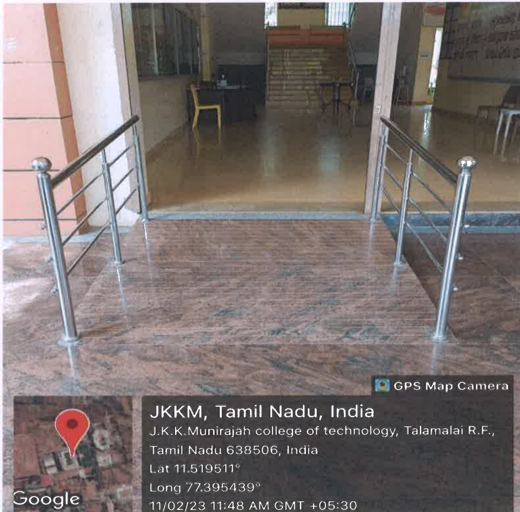
Photos of ramp in main building
