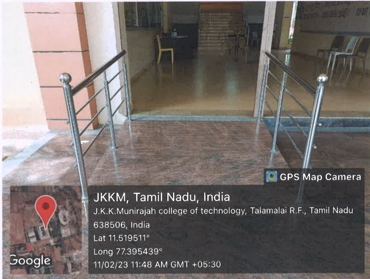
Photos of ramp in main building
