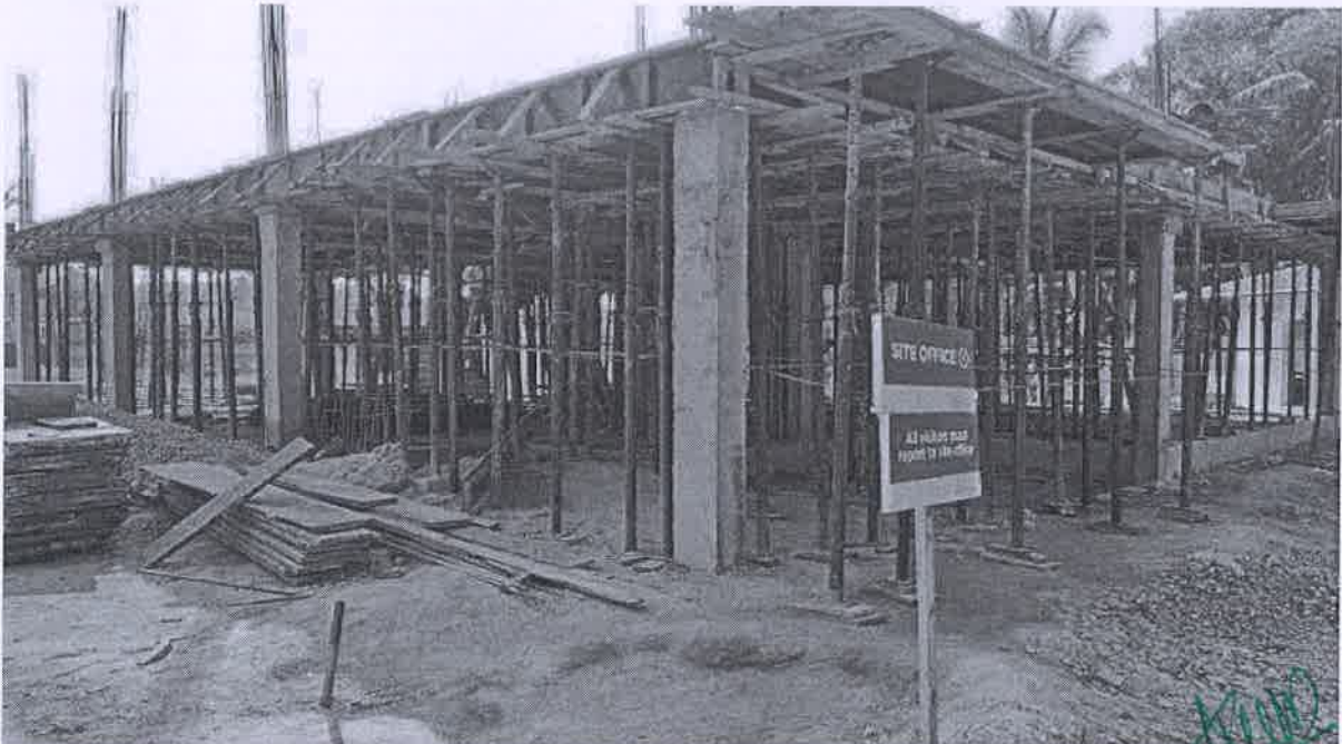
PHOTO OF VISIT AT CHENNIMALAI CONSTRUCTION PLOT AREA
