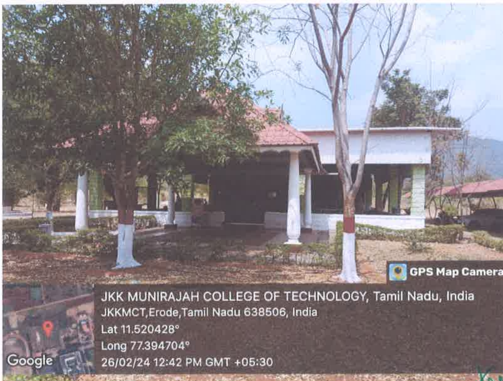
FIG 36: CANTEEN-I OUTSIDE VIEW
