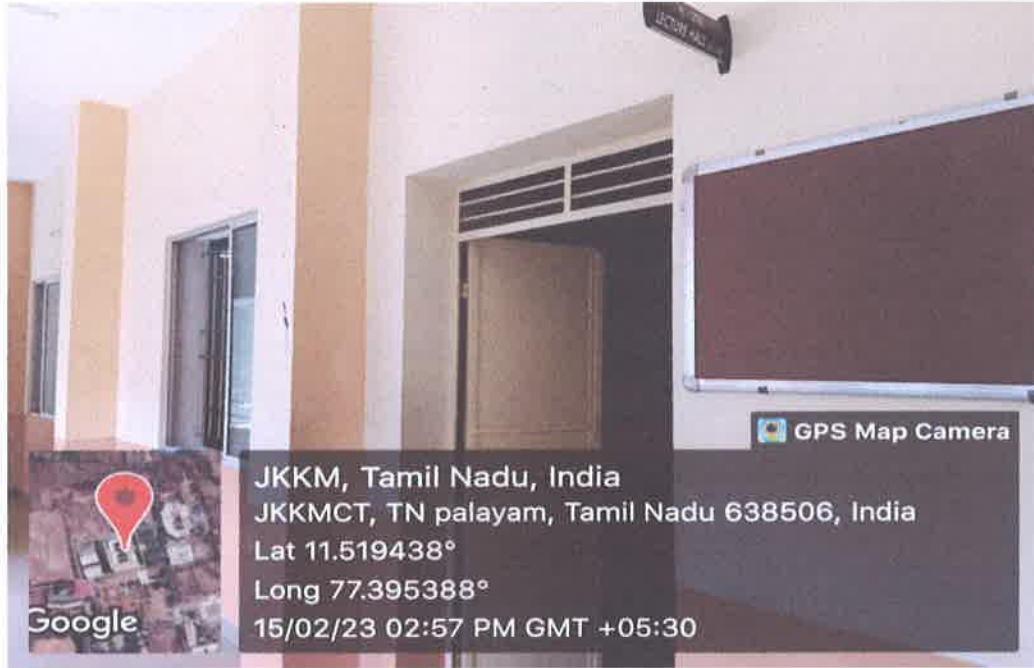
H-202 Classroom outside view
