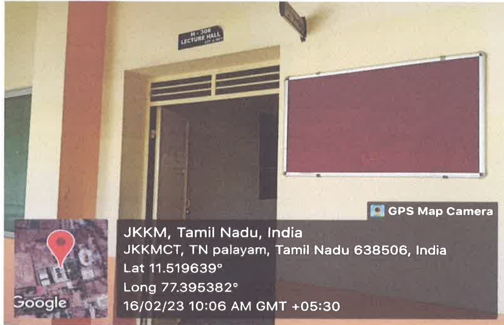
H-306 Classroom outside view
