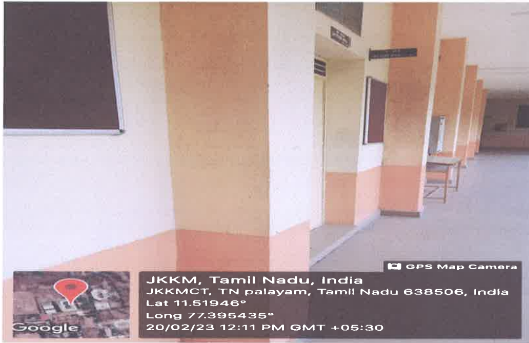
H-414 Classroom outside view
