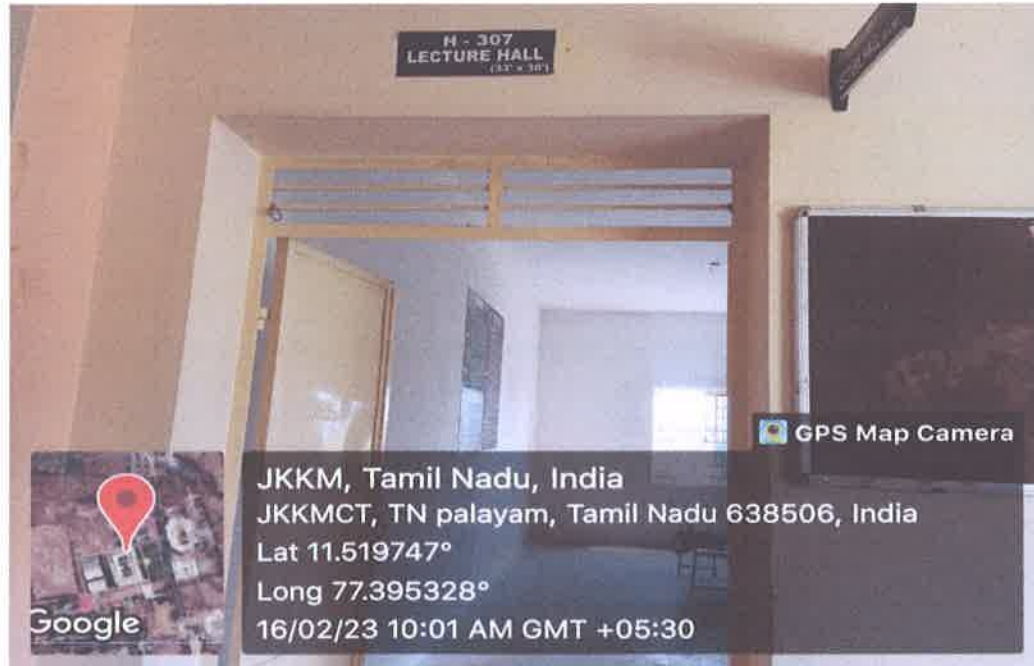
H-307 Classroom outside view
