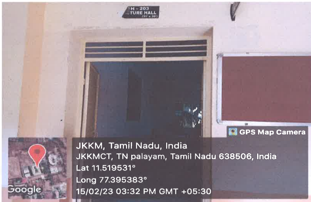
H-203 Classroom outside view
