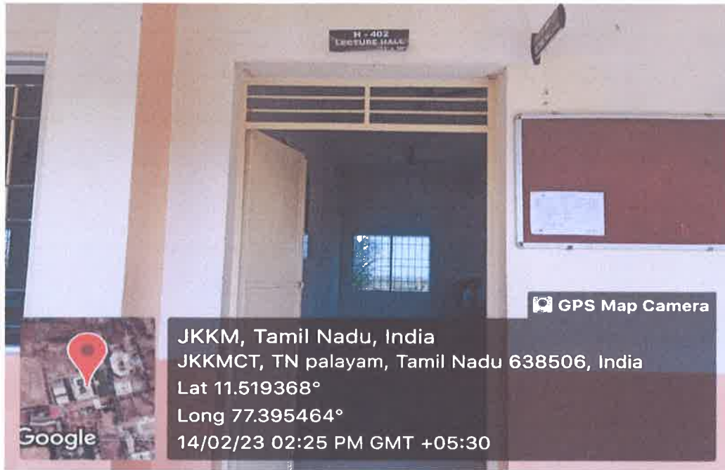
H-402 Classroom outside view
