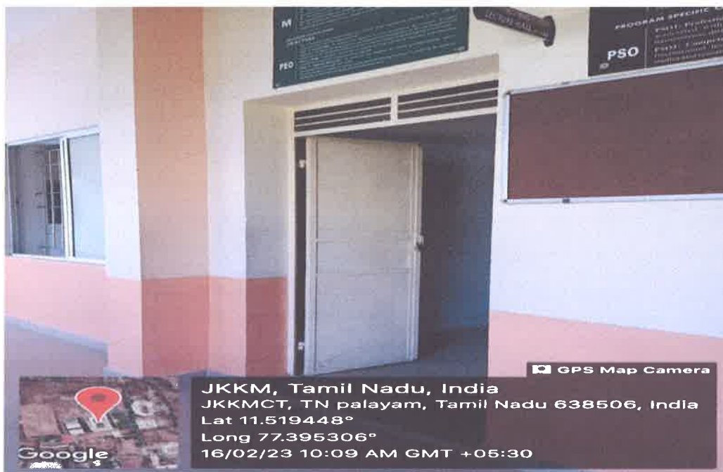
H-305 Classroom outside view
