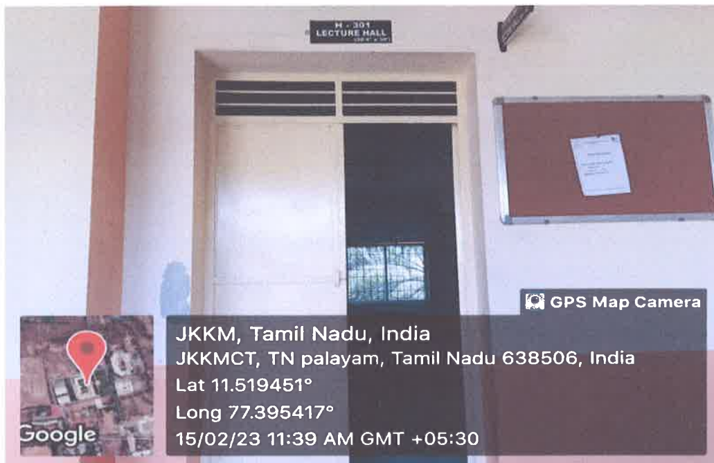
H-301 Classroom outside view
