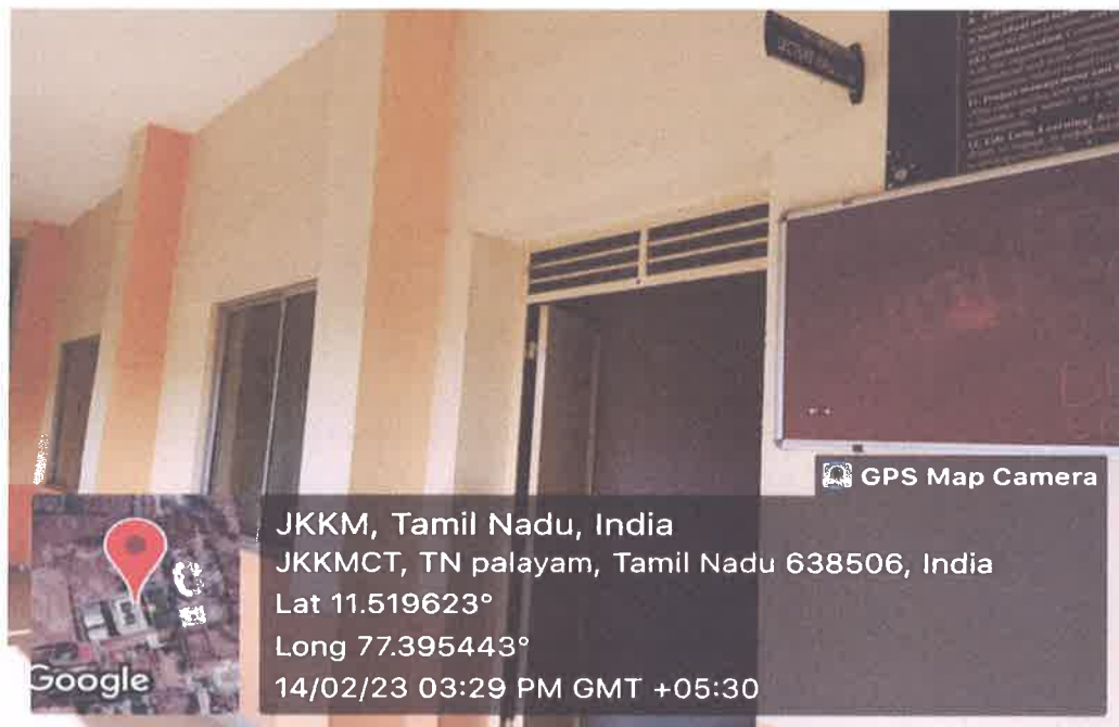
H-410 Classroom outside view
