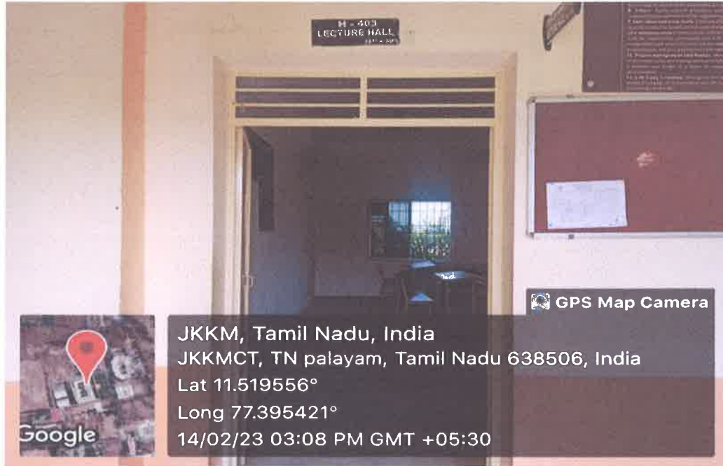
H-403 Classroom outside view
