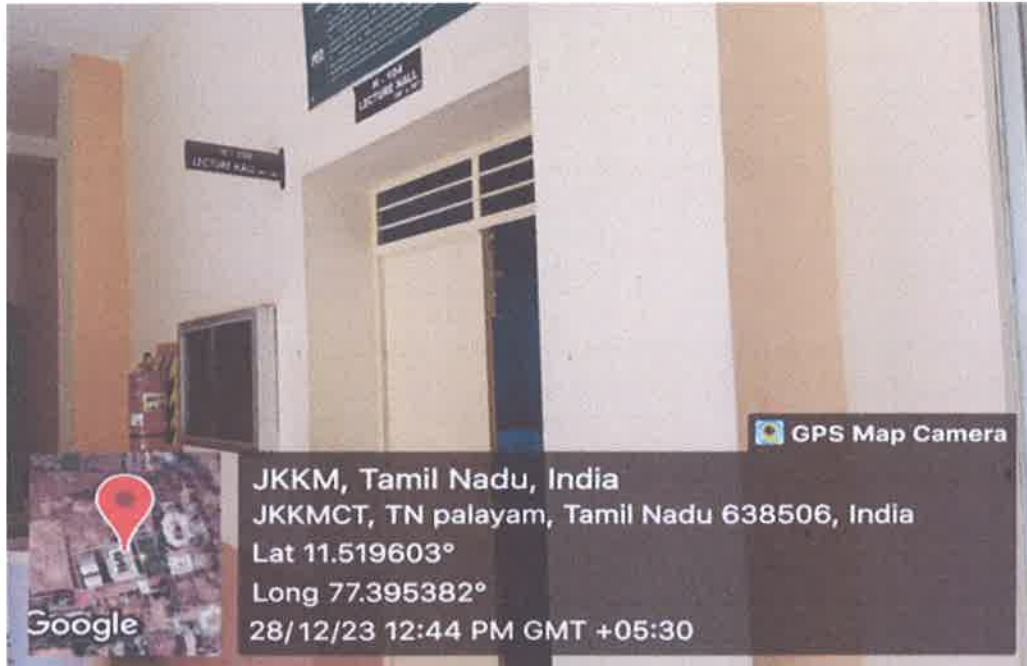
H-104 Classroom outside view
