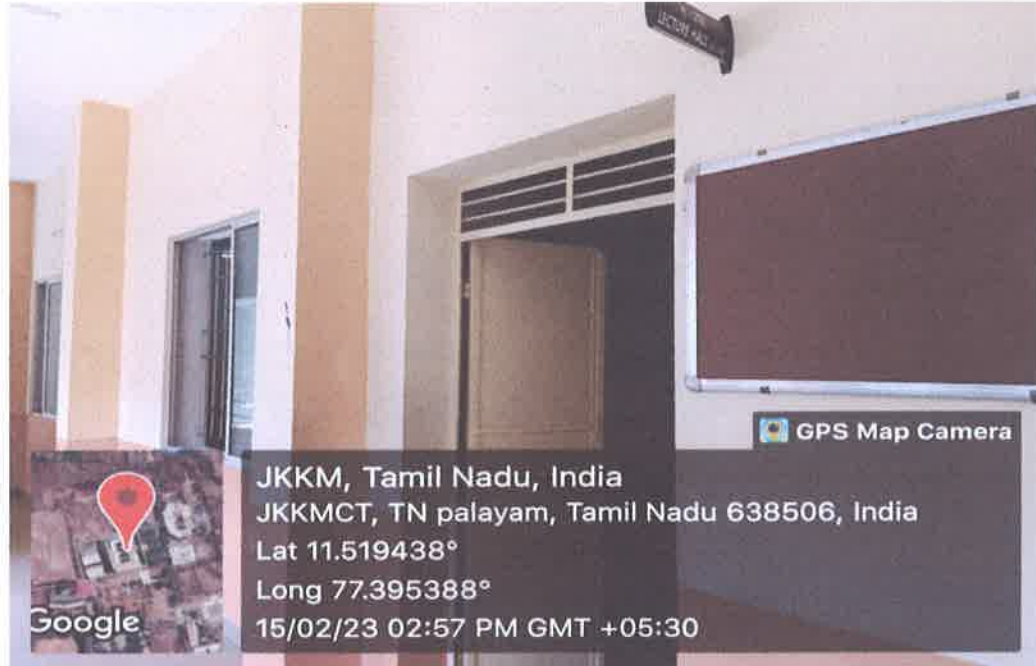
H-202 Classroom outside view
