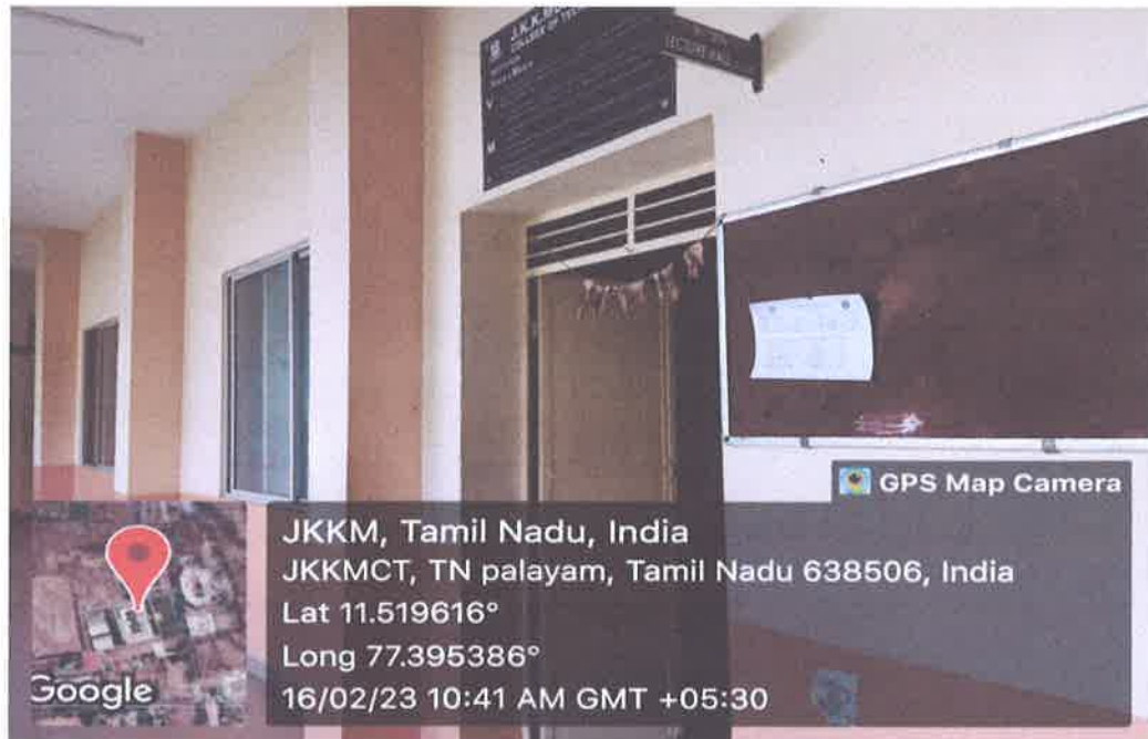
H-206 Classroom outside view
