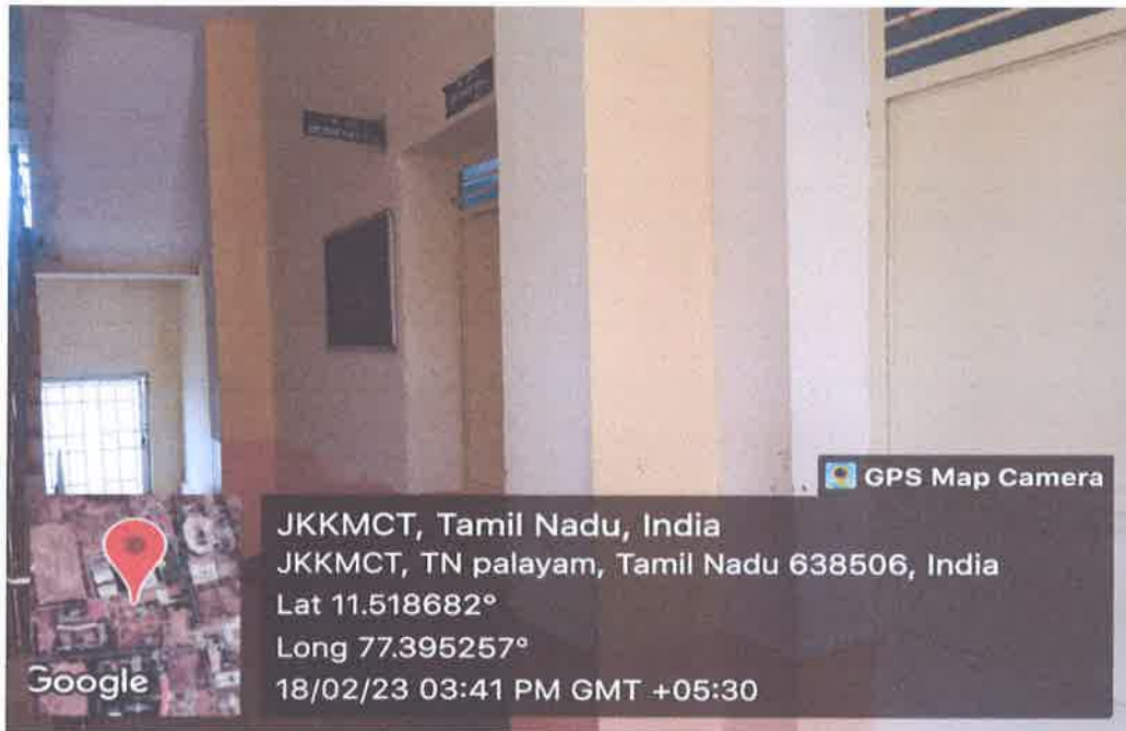
H-412 Classroom outside view
