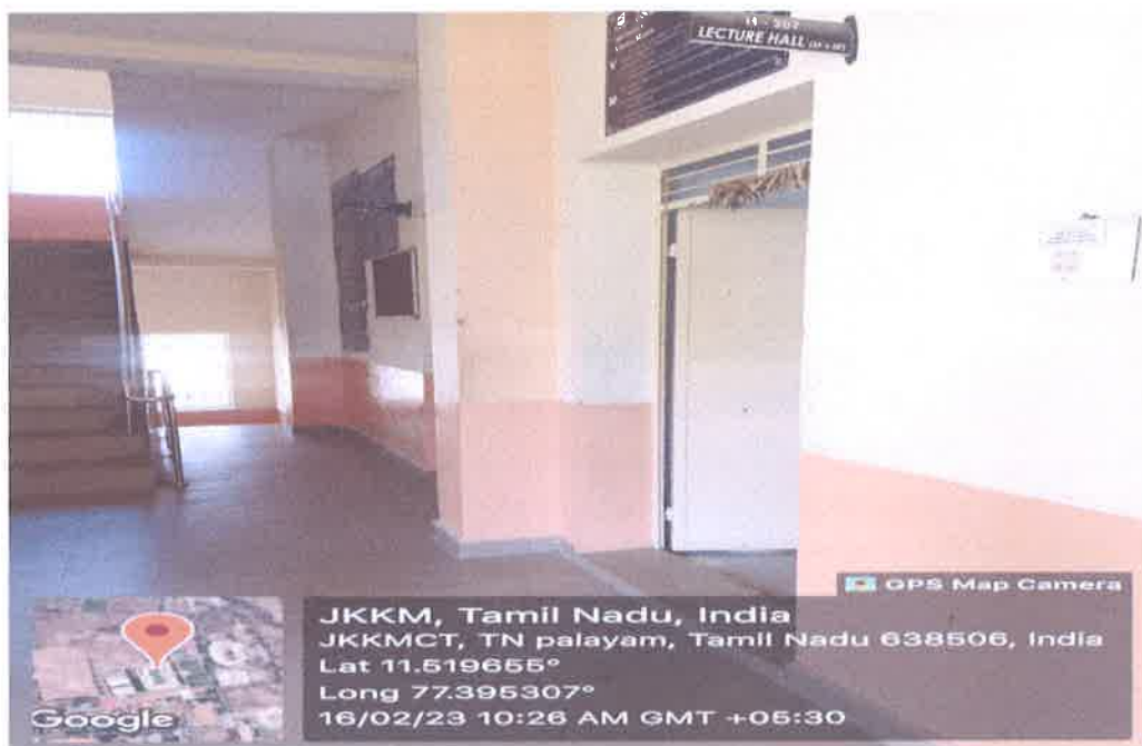
H-207 Classroom outside view
