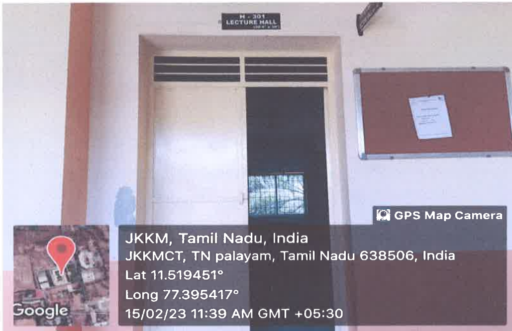
H-301 Classroom outside view
