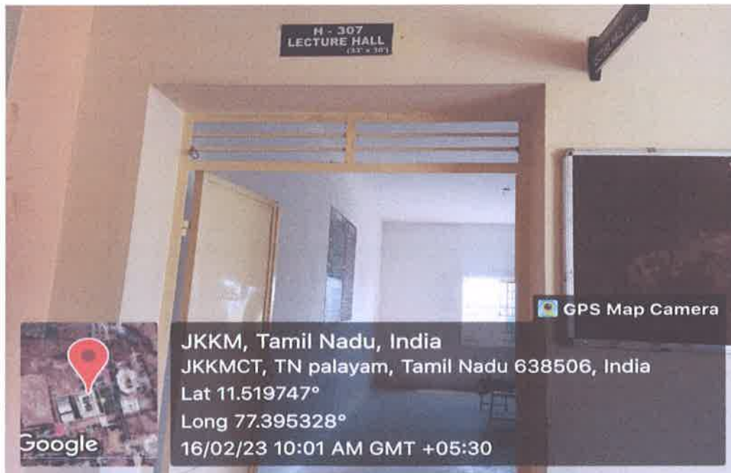
H-307 Classroom outside view
