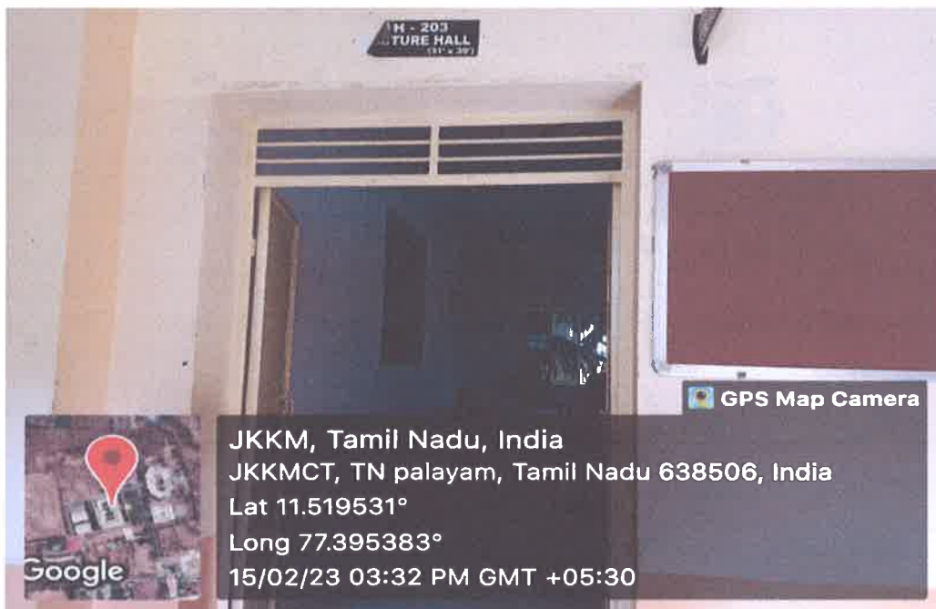
H-203 Classroom outside view
