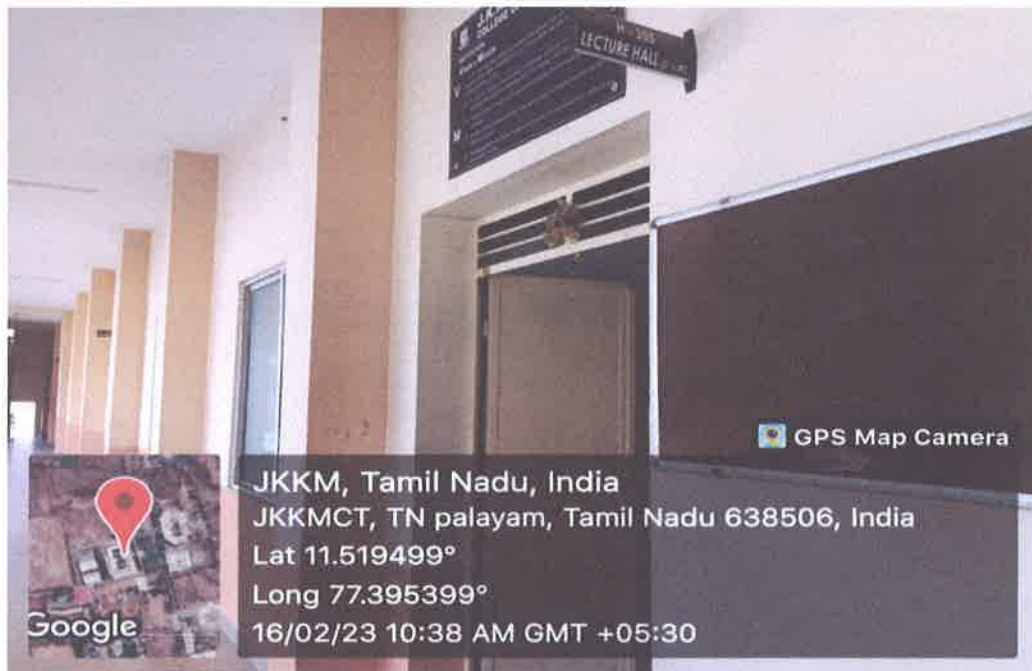
H-205 Classroom outside view
