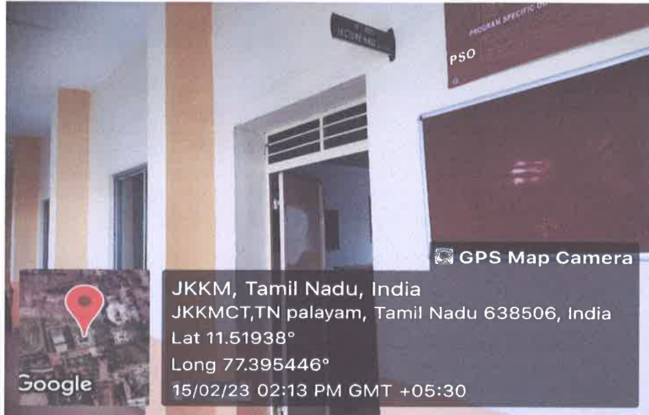
H-420 Classroom outside view
