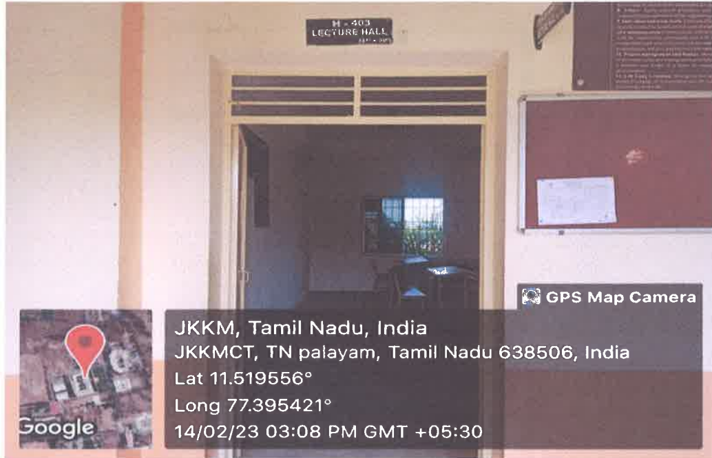
H-403 Classroom outside view
