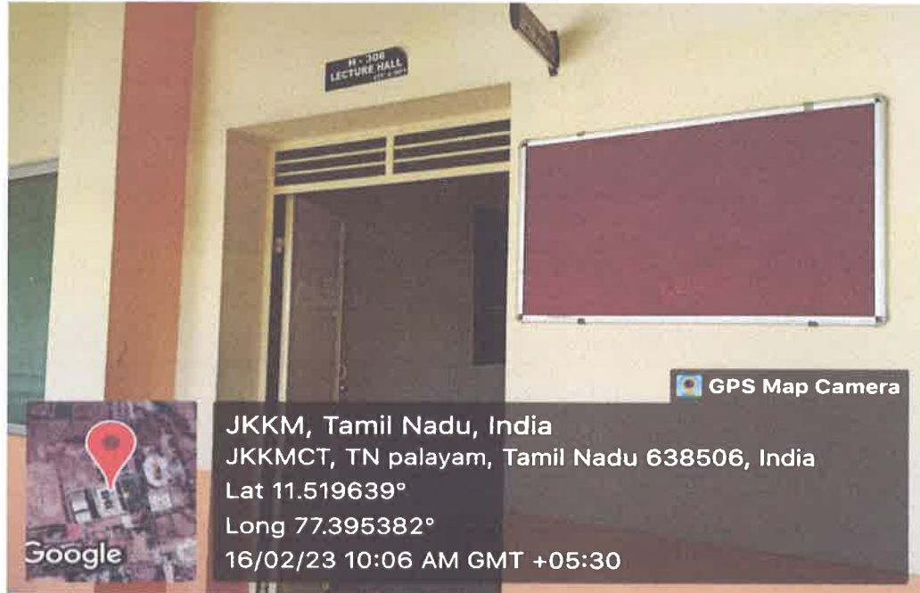
H-306 Classroom outside view
