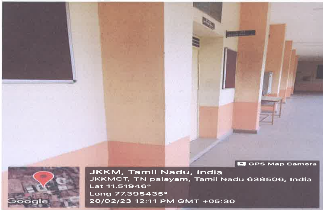
H-414 Classroom outside view
