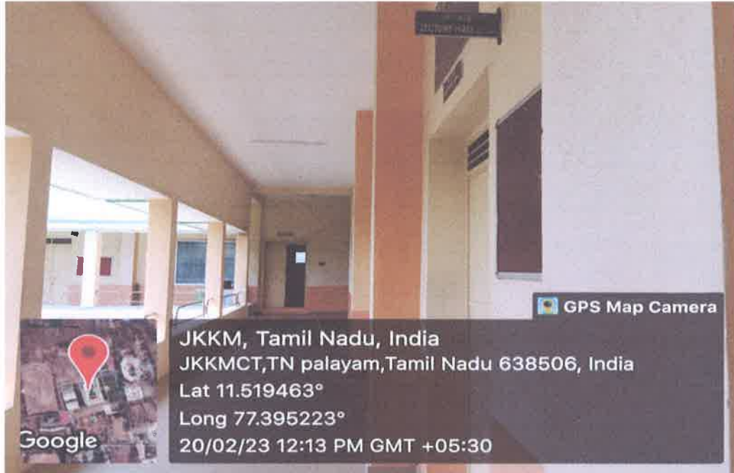
H-415 Classroom outside view
