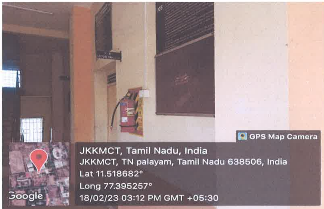
H-411 Classroom outside view
