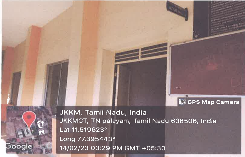
H-410 Classroom outside view
