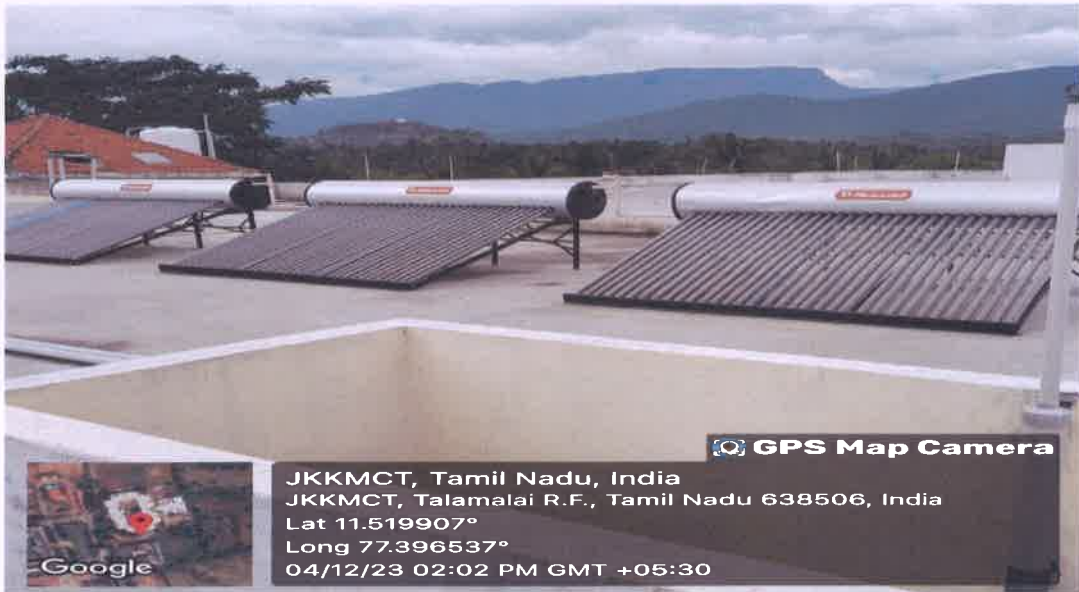
Photos of Solar Water Heater located at Boys Hostel
