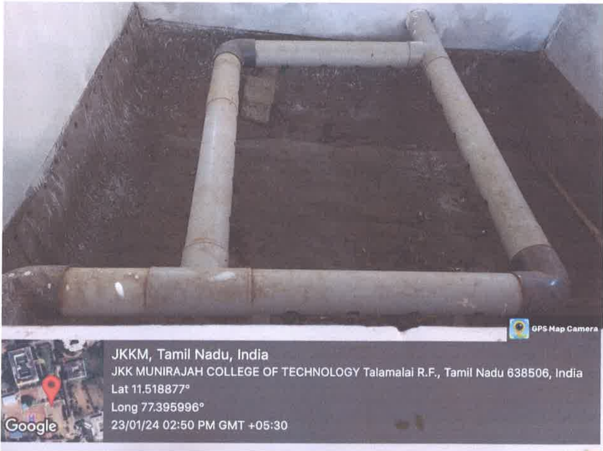
Photos of inside view of Rainwater Harvesting Structure
