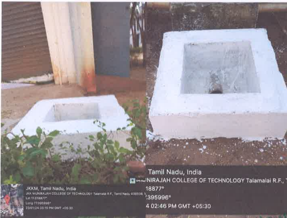
Photos of Rainwater Harvesting Chamber
