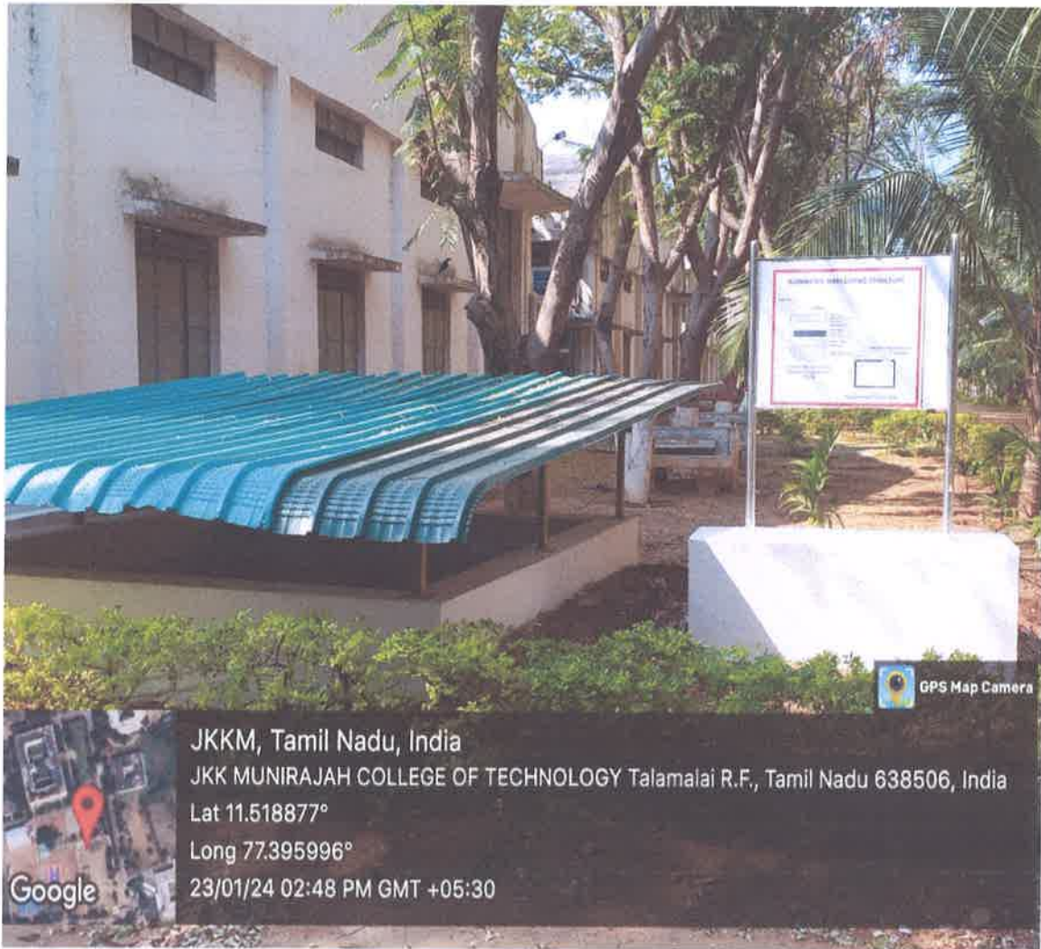
Photos of Rainwater Harvesting Structure
