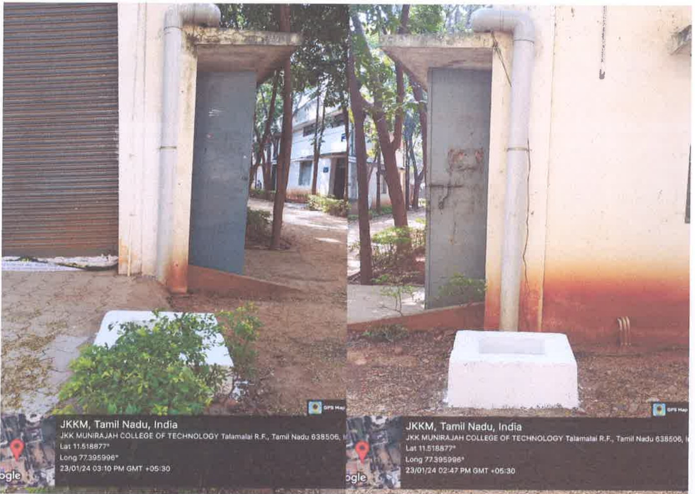
Photos of Rainwater pipe lines
