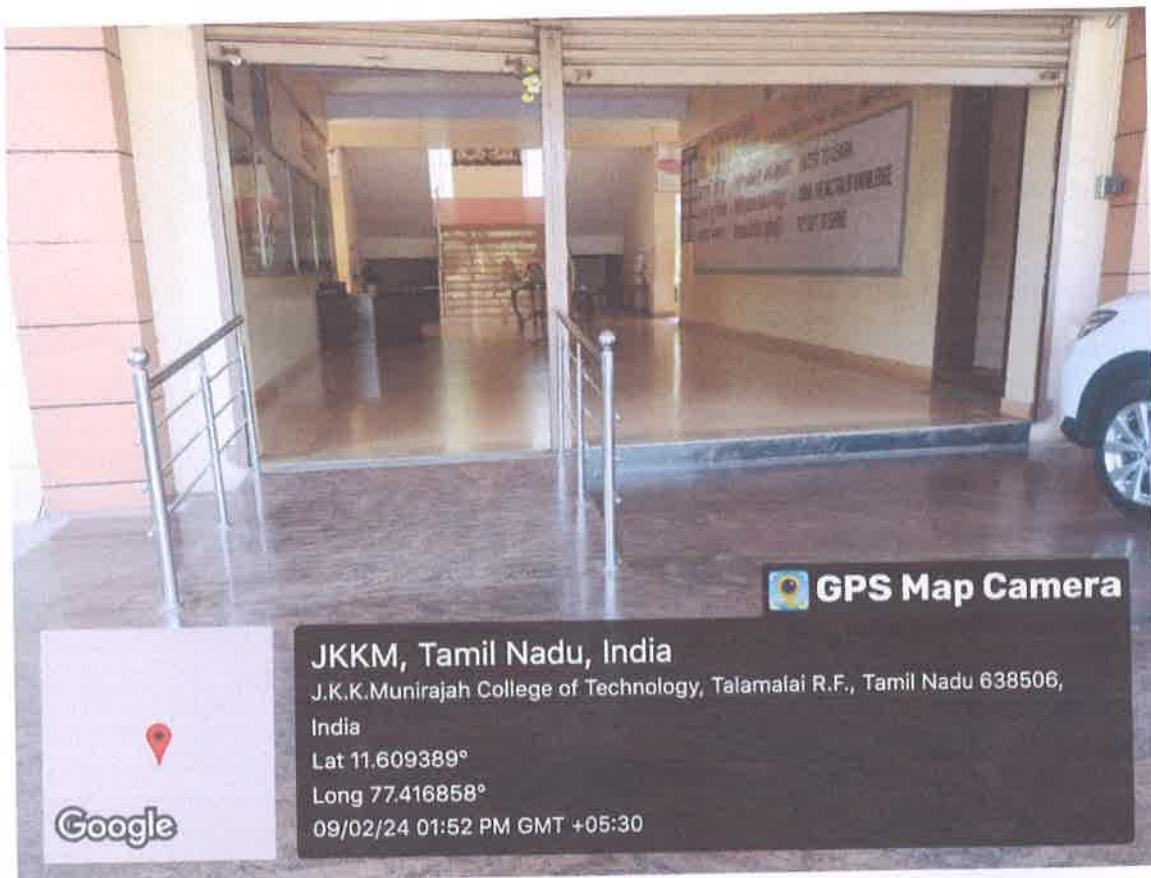
Photos of ramp in main building
