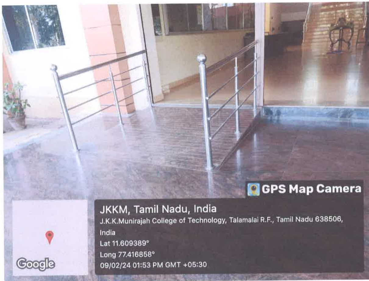
Photos of ramp in main building
