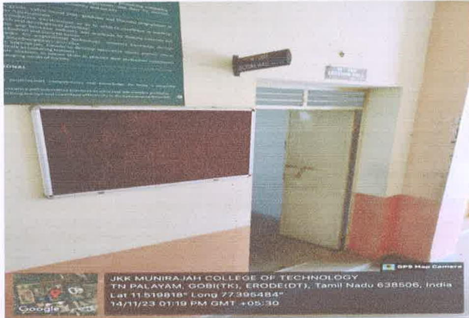
H-208 Classroom outside view
