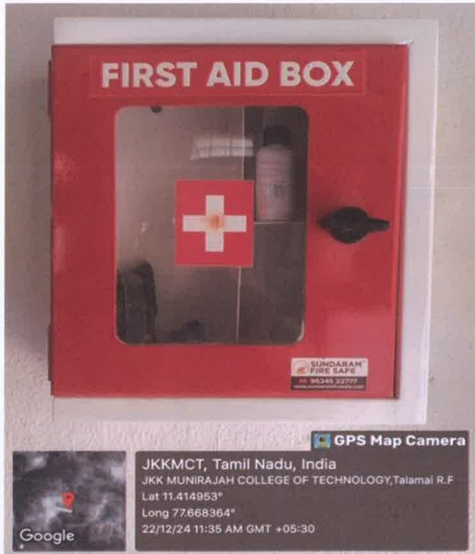
Photo of First aid box fixed in Floor & all laboratories
