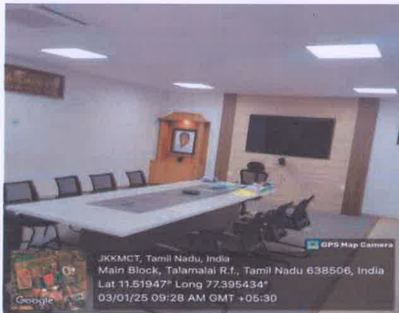
Photos of sensor-based AC in our college Board room
