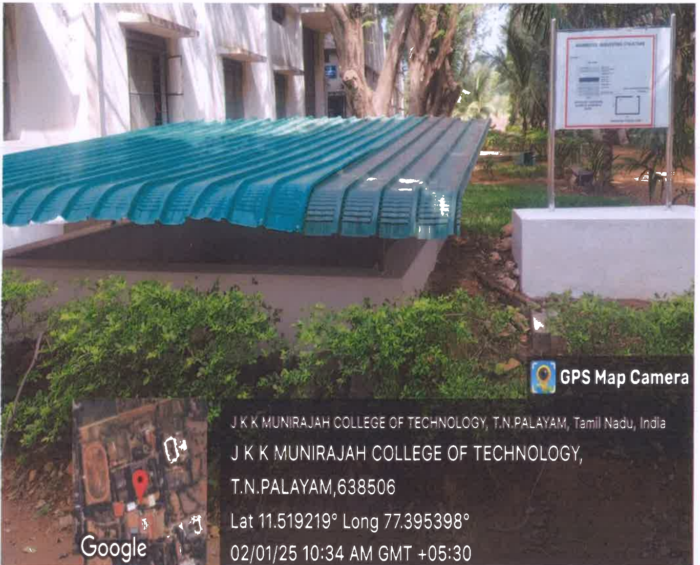
Photo of Rainwater Harvesting Structure
