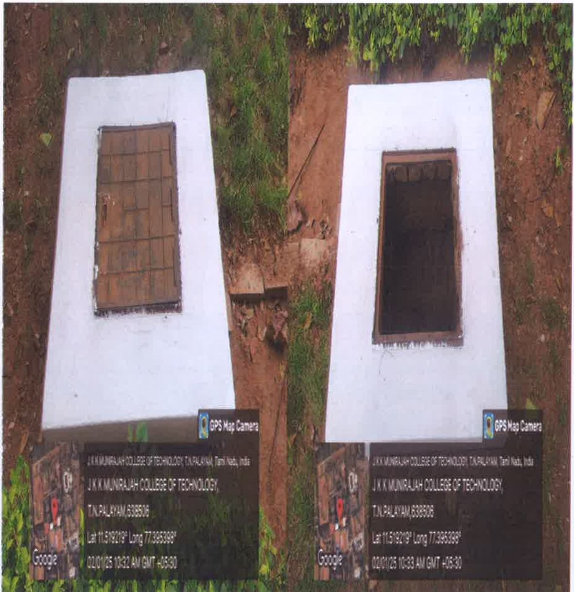
Photo of Tanks and Bunds
