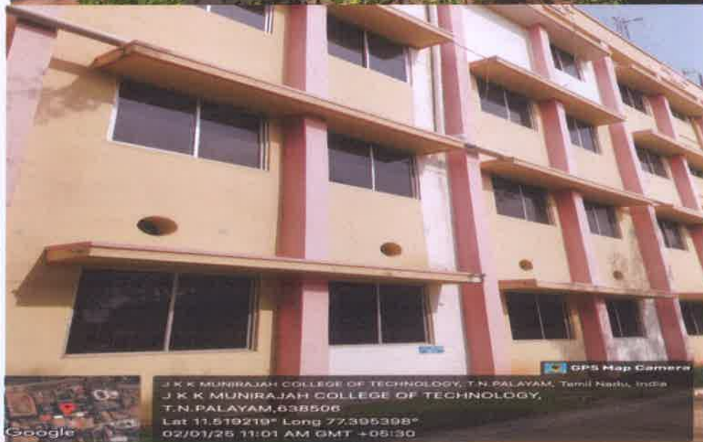
Photo of Rainwater pipe lines in Main Block
