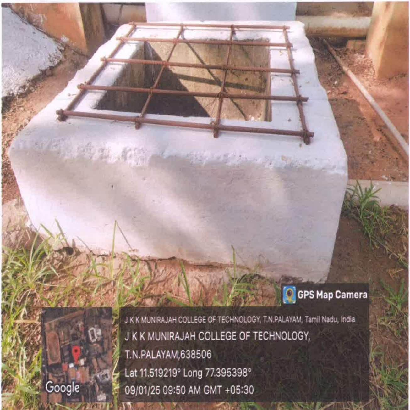
Photo of Rainwater Harvesting Chamber
