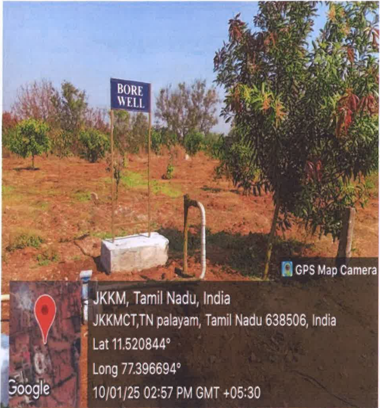
Photo of Bore Well in Boys hostel
