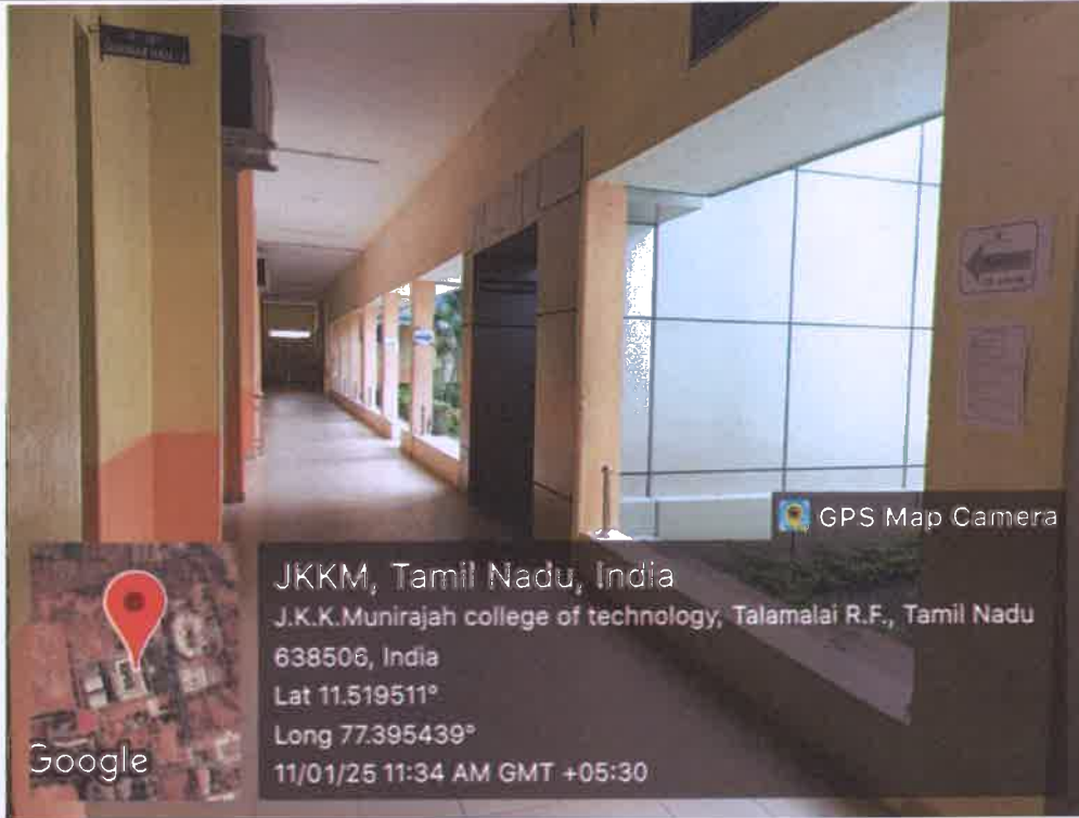
Photos of way to lift from the corridor
