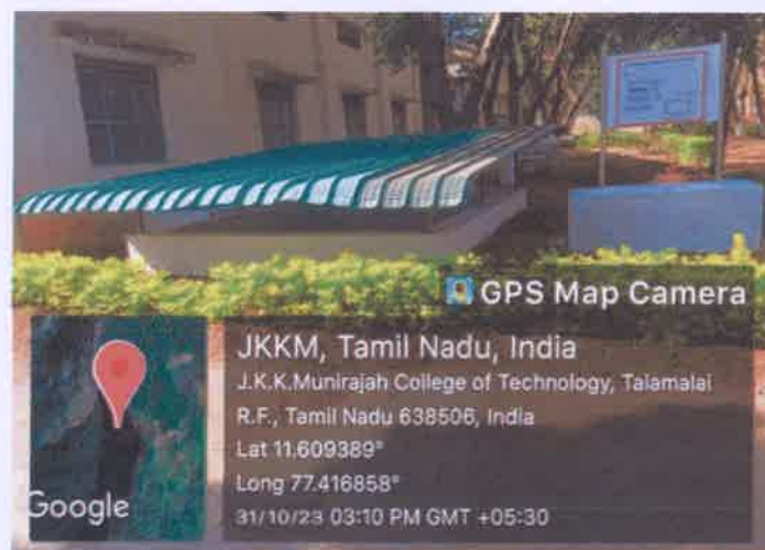
Photos of Rain Water Harvesting structure
