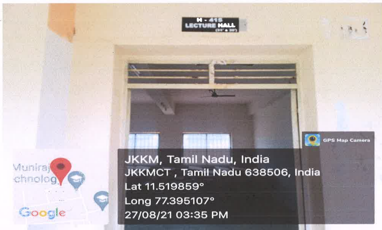
H-415 Classroom outside view
