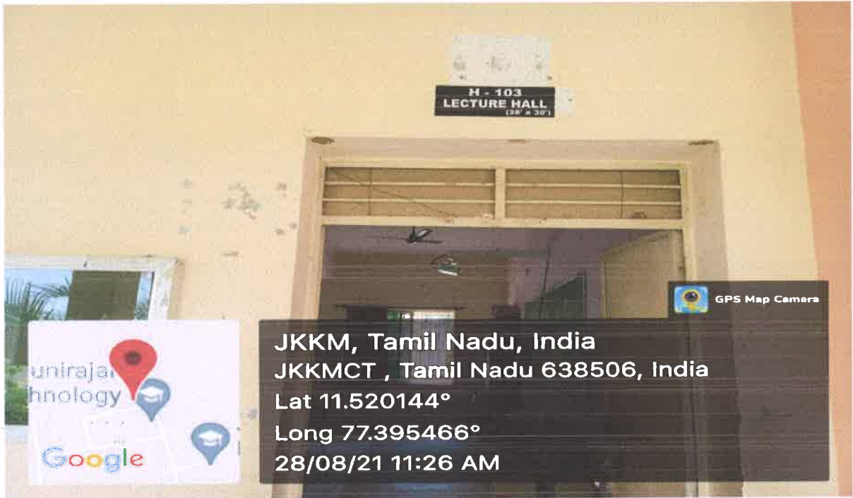
H-103 Classroom outside view
