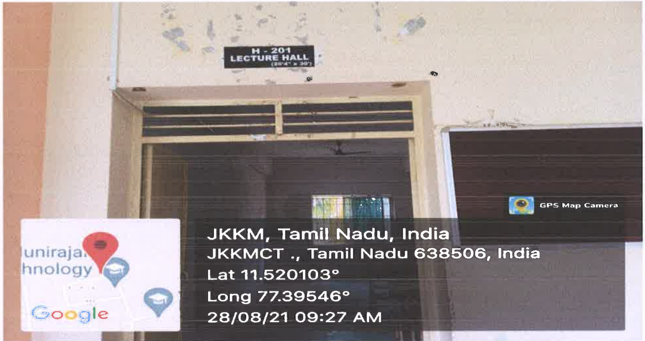
H-201 Classroom outside view
