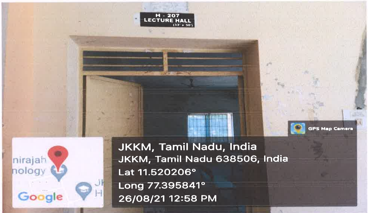
H-207 Classroom outside view
