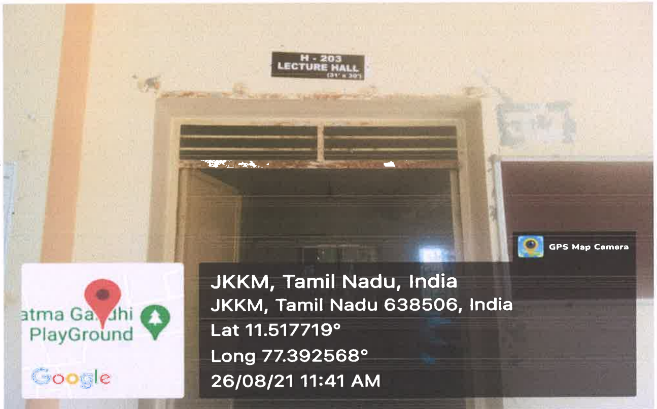
H-203 Classroom outside view
