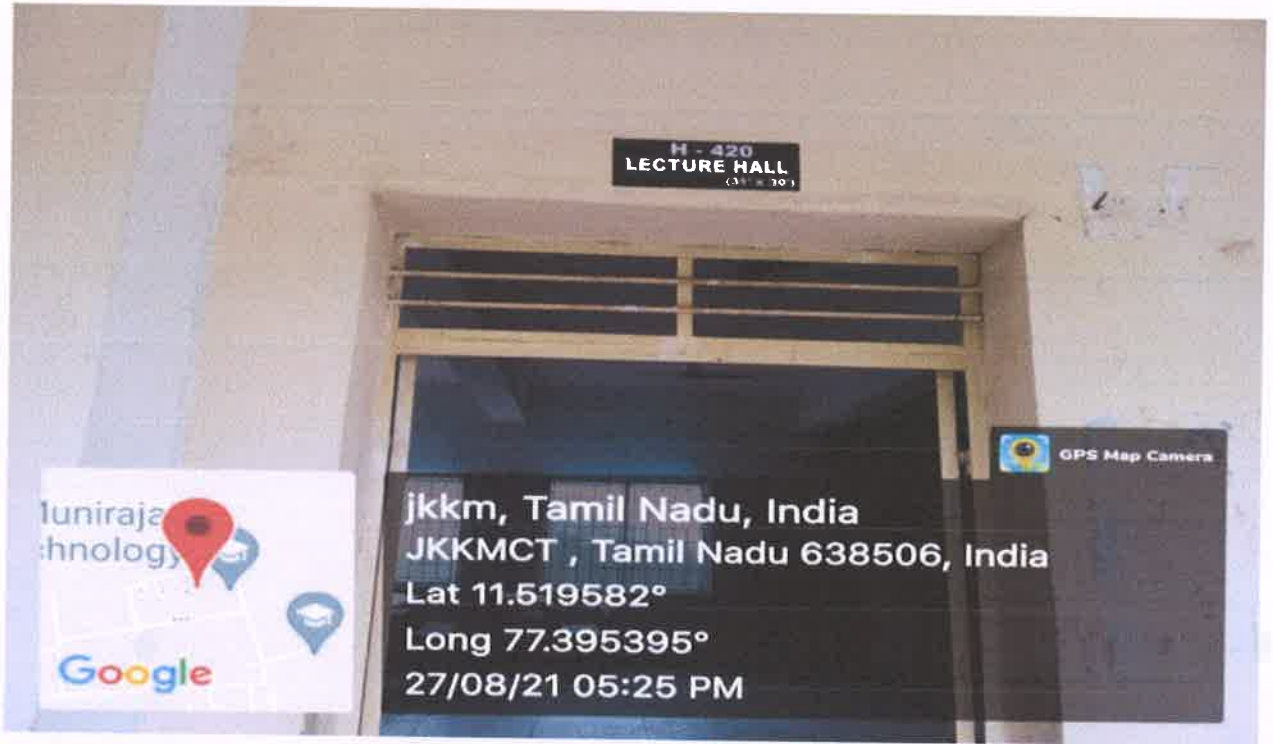
H-420 Classroom outside view
