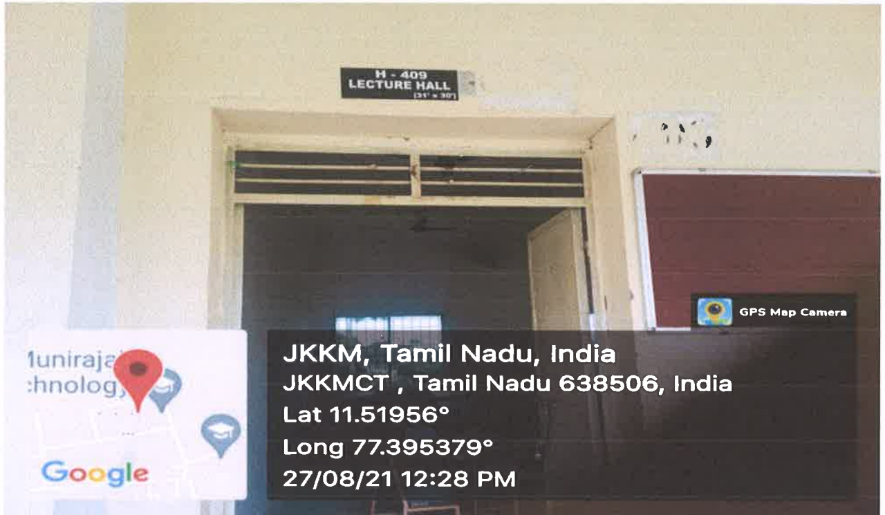
H-409 Classroom outside view
