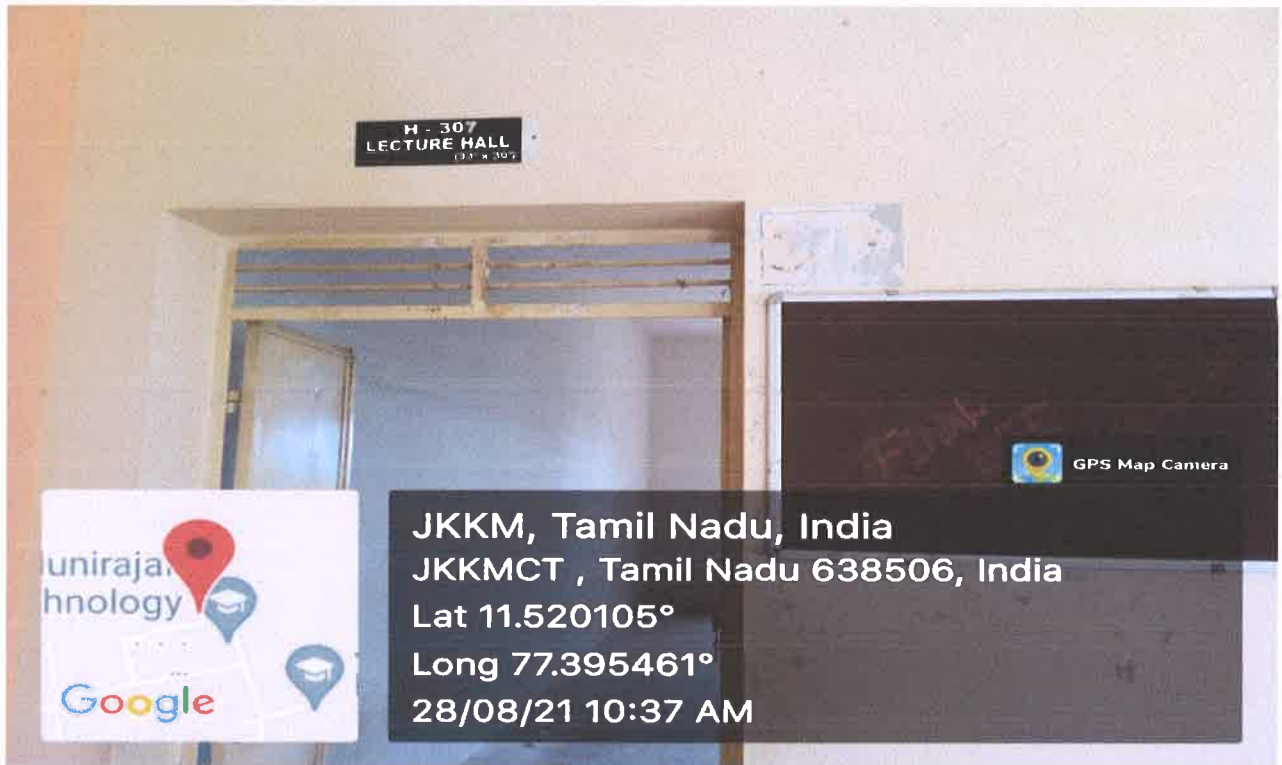
H-307 Classroom outside view
