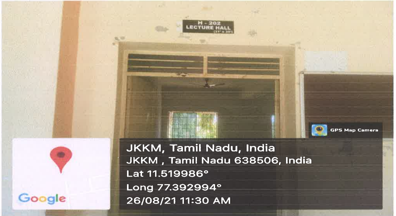
H-202 Classroom outside view
