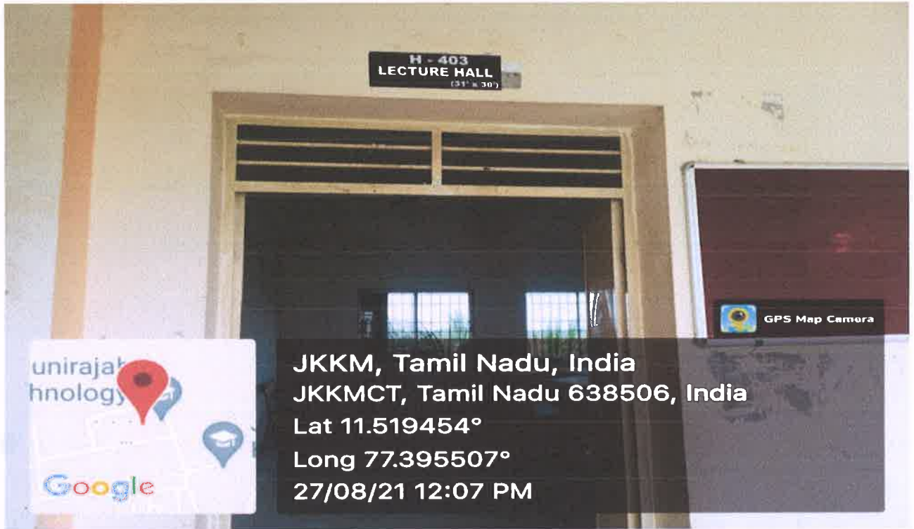
H-403 Classroom outside view
