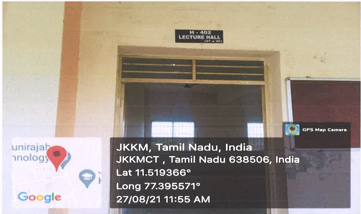
H-402 Classroom outside view
