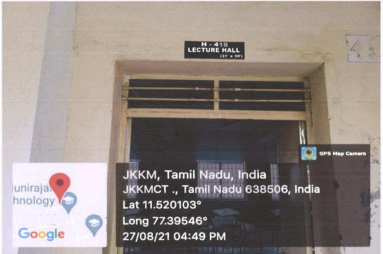
H-418 Classroom outside view
