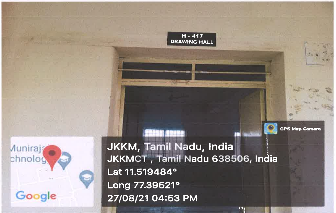
H-417 Classroom outside view
