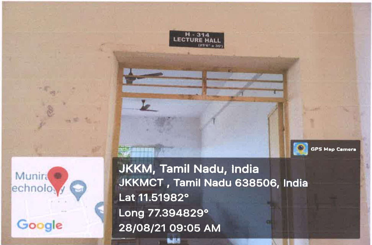
H-314 Classroom outside view
