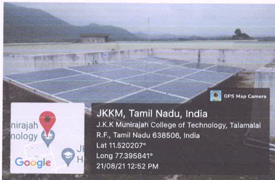
Solar Plant Located at Our Main Building Roof-Top
